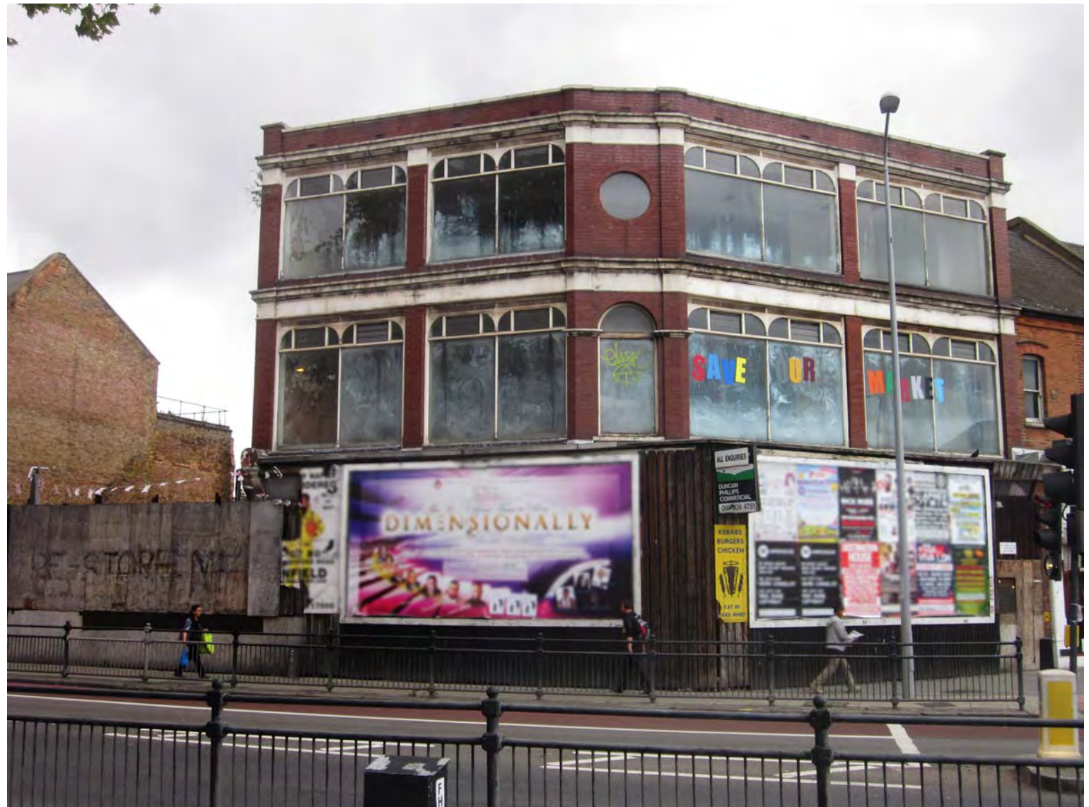
Figure 41 Picture of the corner building as it lays now, unused
