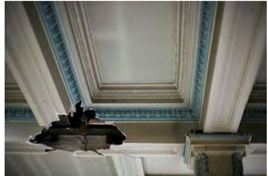
Figure 50 Existing cornice on first floor
