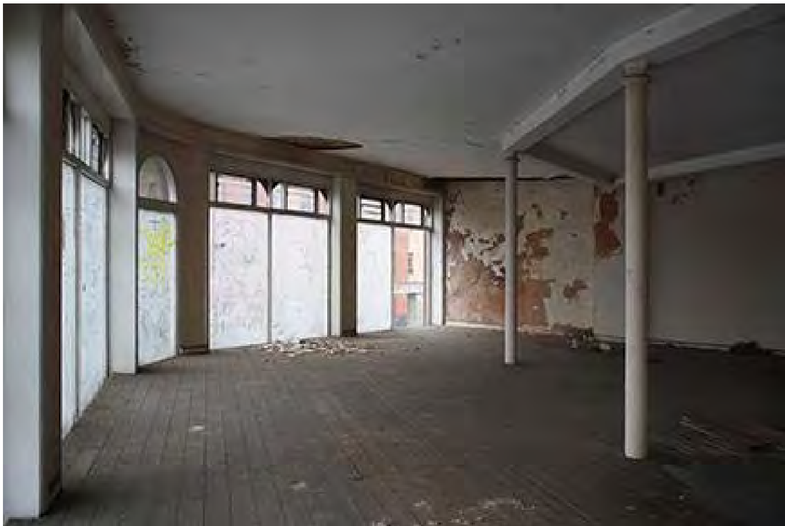
Figure 1 Inside the corner building at Wards Corner
