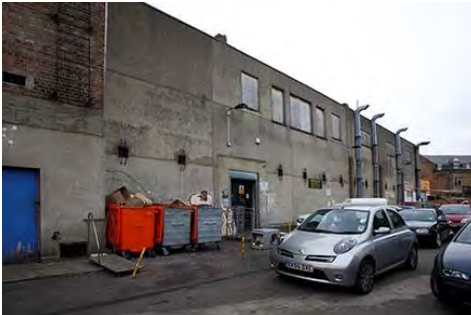
Figure 48 View of the rear of building
