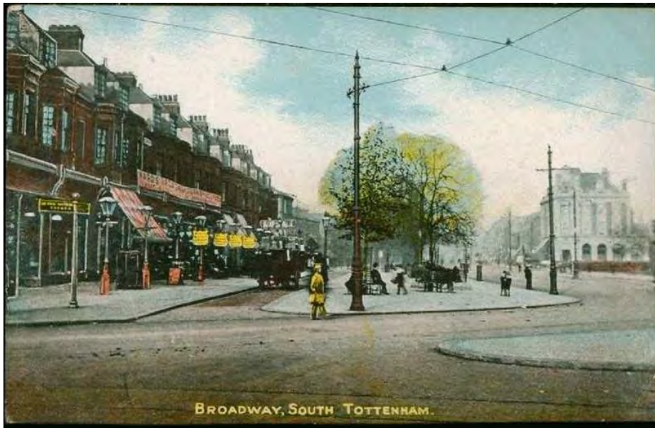
Figure 53 Old photo showing bays, dormers, original frontages and chimneys now removed
